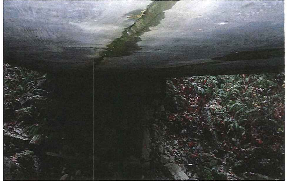
CK2138 Abutment Left Bank
