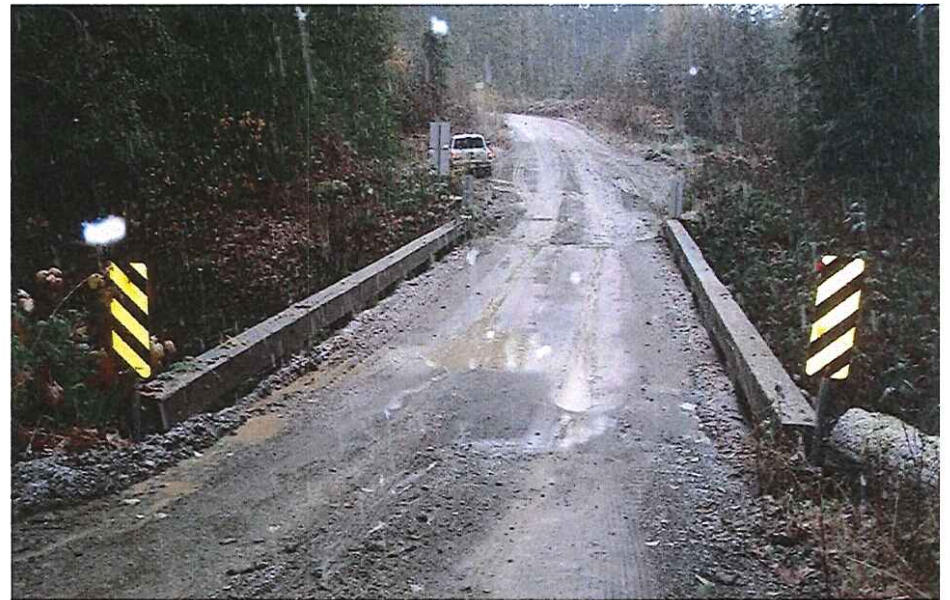
CK2138 Approach Right Bank
