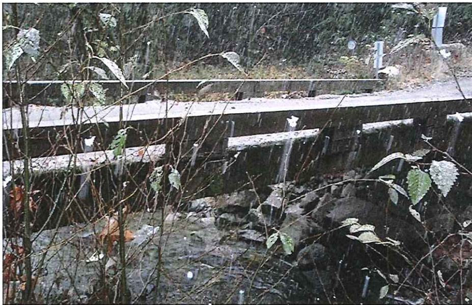
CK2138 Crossing Upstream
