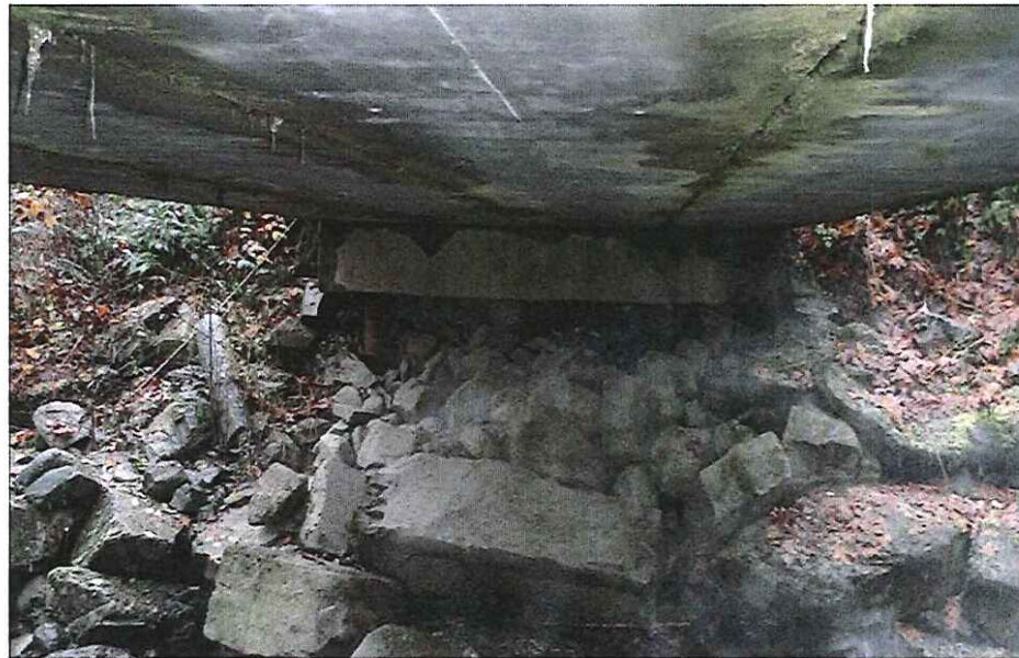
CK2138 Abutment Right Bank
